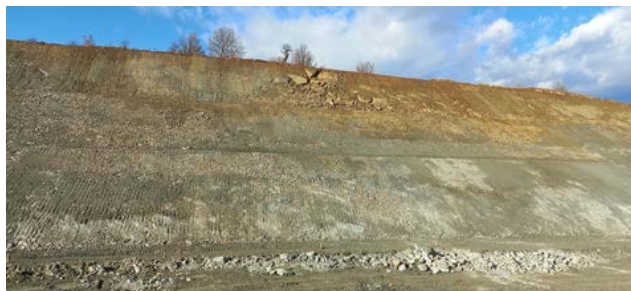
Figure 2 The initial stage of the rockslide (01.02.2023).
