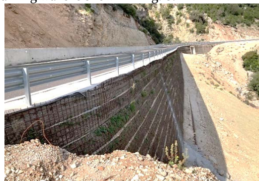
Figure 8 GRS retaining wall (Huesker).
