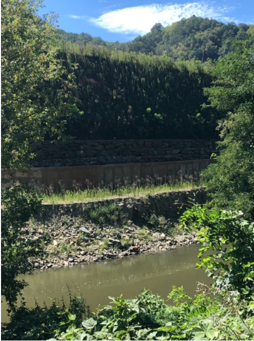
Figure 7 Finished RSE with green facing
