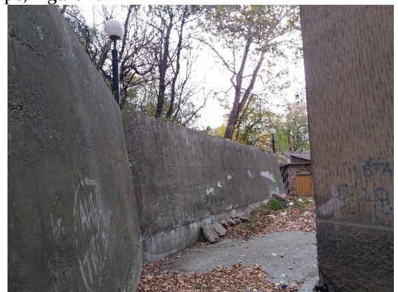
Figure 1. A section of the existing retaining system at the slope toe
