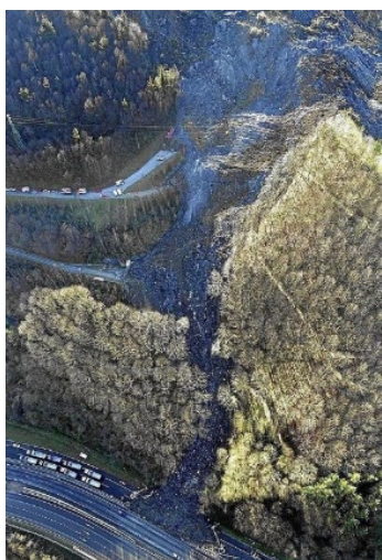
Fig 1. The Landslides slope
