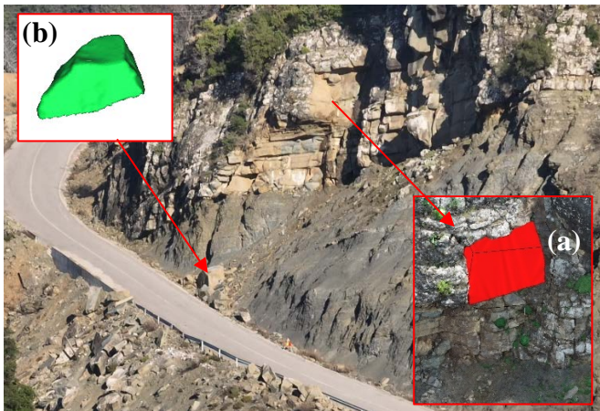
Figure 8 The northern section of the slope clearly reveals the origin of rockfalls in Type III flysch above Type VIII. The failure mechanism is evident, characterized by the undercutting of the sandstone as a result of the differential erosion of the underlying siltstone. a) the main rockfall source with 13 m 3 volume, measured by digital reconstruction of the detachment geometry, and b) a 6.5 m 3 block from this detachment, located on the slope side.
