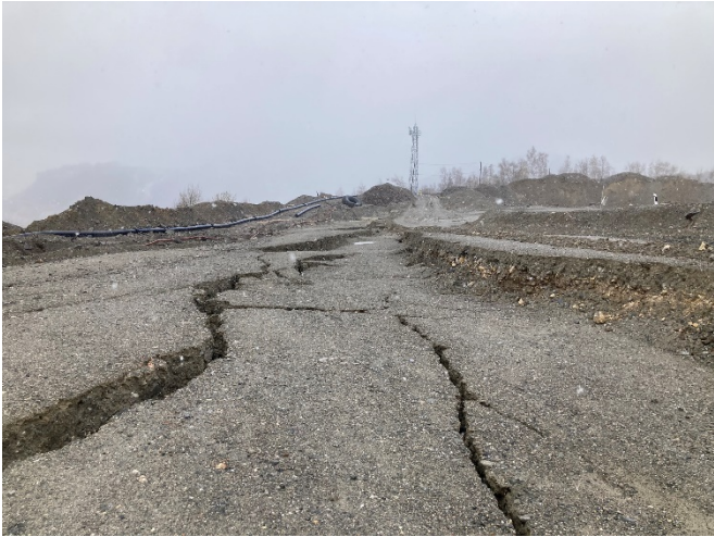
Figure 2 Gaping cracks and local benching between conjugated failure planes on the abandoned tailing horizon 550 m.
