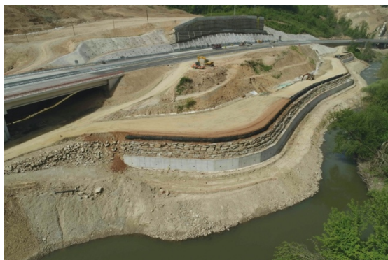
Figure 2 Alignment of the RSE on top of protective structure
