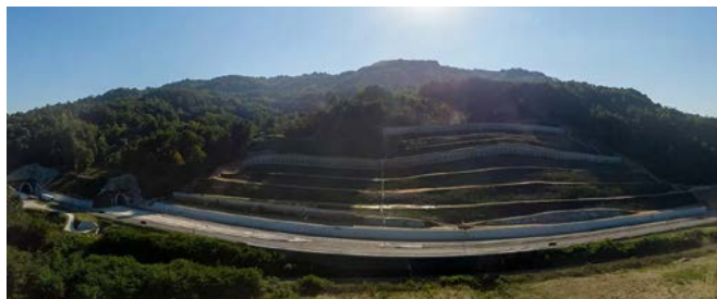
Figure 16 Landslide remediation
