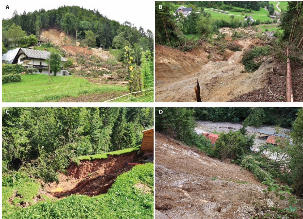
Figure 6 Examples of slope mass movements. A) Landslide that has mobilised into a debris flow, consisting of sand, gravel and several boulders with a size of several m 2 . B) At the bottom of the valley, the debris flow has partially covered the stream bed. C) An example of a landslide that has mobilised into a mudslide of sand, silt and clay. D) An example of a water-saturated slide with roots and trees that led to the complete destruction of a house. The landslide occurred on a limestone base, which is unusual for landslides to occur.
