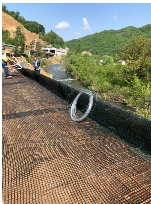
Figure 7 Installation of geosynthetic materials
